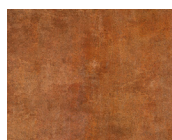
FCR 504 535 Thick rust
